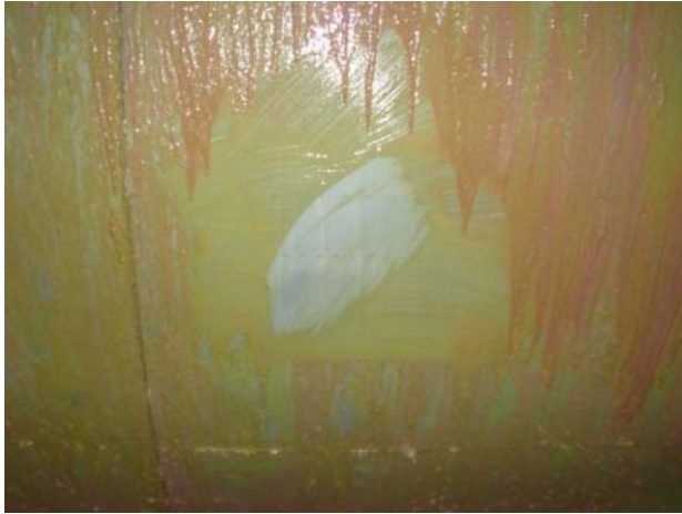
Image 3: 12:00pm inspection release of primer is noted waited until 2:30 for pressure rinse
